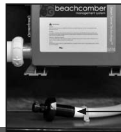
Drain / Fill Valve
